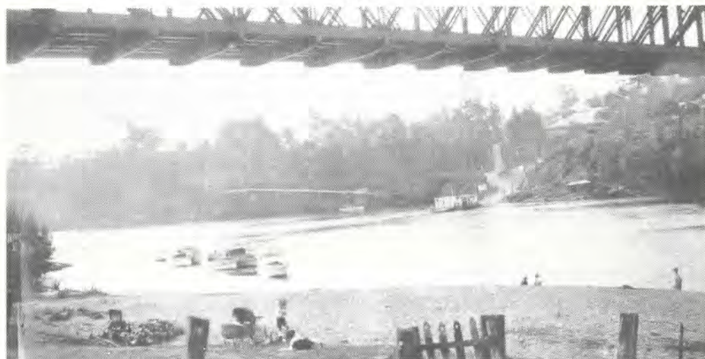
The Sand Patch on the far side of the river, under the railway bridge. The vehicular ferry crossing the river.
