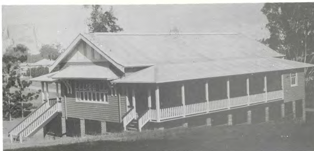
Holy Family church/school, Indooroopilly, building blessed and opened on 4th July, 1926.
