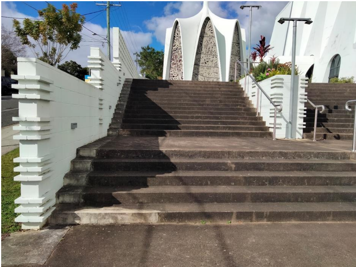
Fig 4 New Retaining Wall, Central Garden and Lighting
